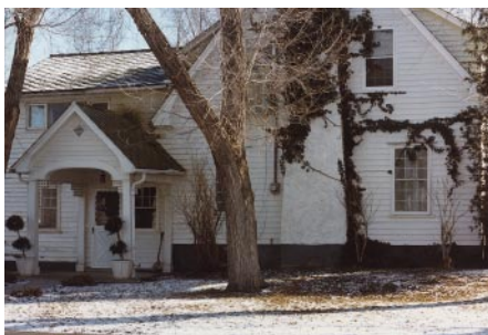
The Wallins two story addition at the back of the house and a pretty back porch.
